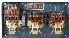
Interior View of MK2 FASD
