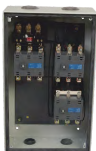
Interior View of ML SASD
