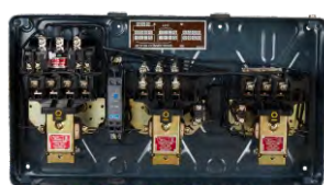
Interior View of MK1 FASD
